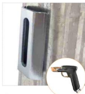
1. Weld the bend plate to the gate jamb 焊接折弯板到门框边框
